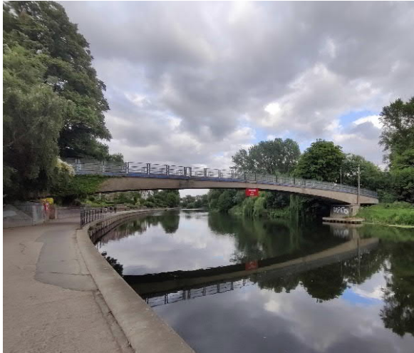
Figure 3-51 - Castle Walk Footbridge
