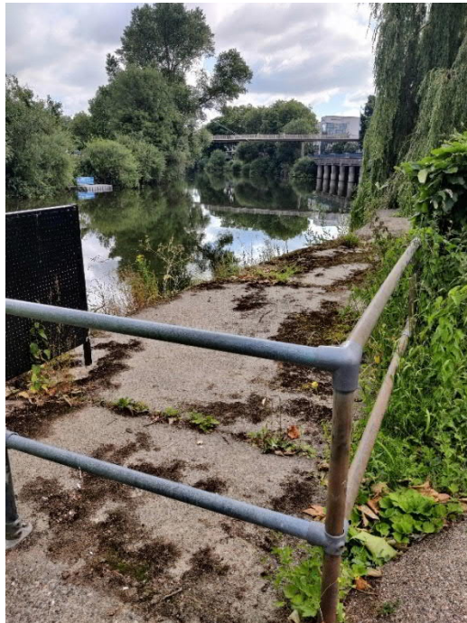
Figure 3-16 - Metal railings at the eastern end of the metal barrier
