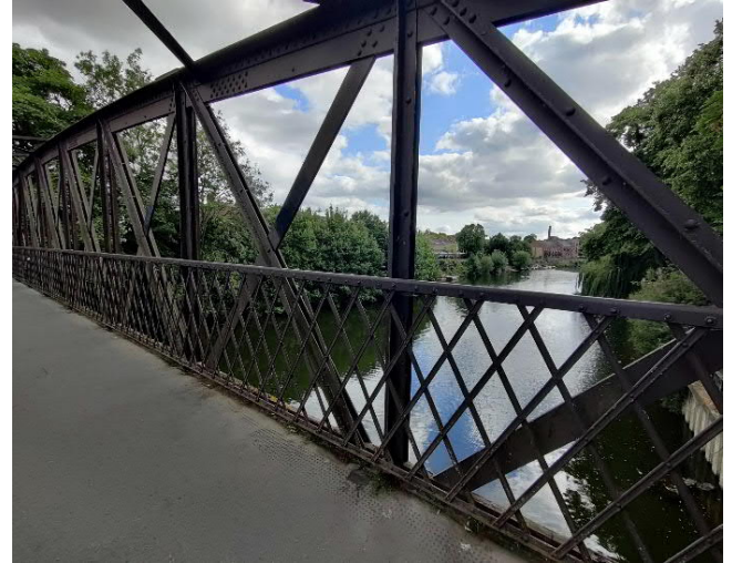
Figure 3-49 - Greyfriars Bridge parapet
