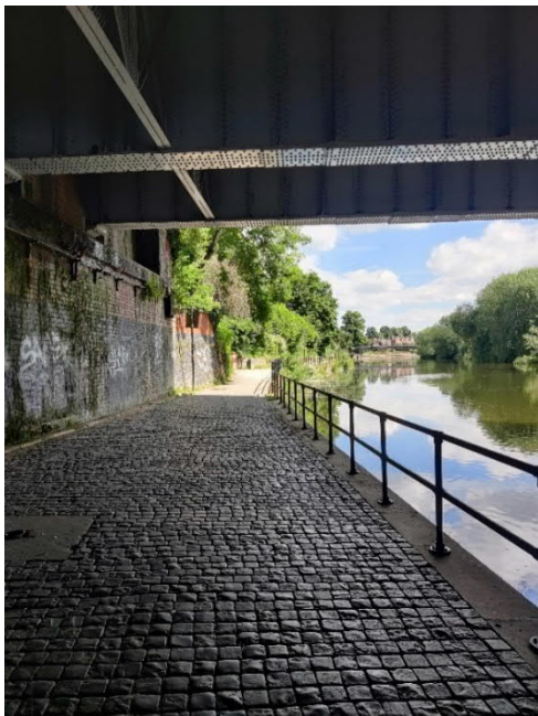
Figure 3-39 - Cobbled stones under railway bridge
