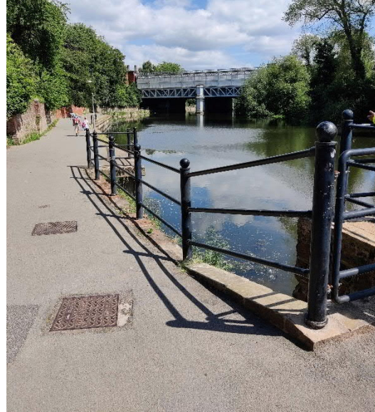
Figure 3-38 - Railings at St. Mary's Water Lane
