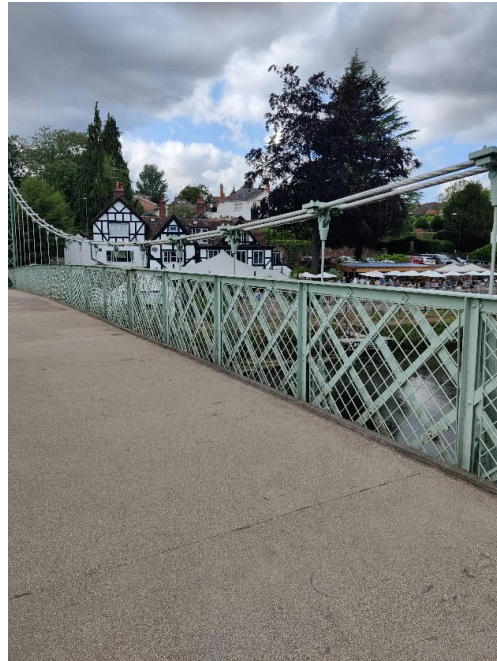
Figure 3-45 - Porthill Bridge parapet
