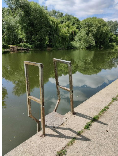
Figure 3-67 - Ladder at the weir
