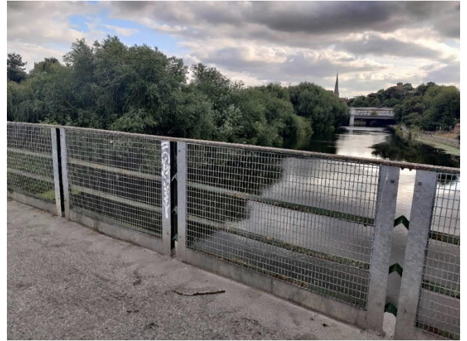
Figure 3-52 - Castle Walk bridge parapet
