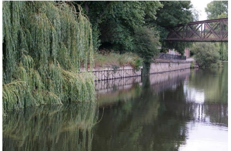
Figure 3-32 - River's edge adjacent to Greyfriars Bridge
