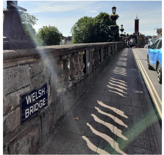
Figure 3-43 - Welsh Bridge balusters
