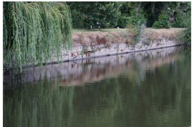
Figure 3-30 - River's edge adjacent to path
