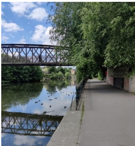
Figure 3-33 - Path below Greyfriars Bridge
