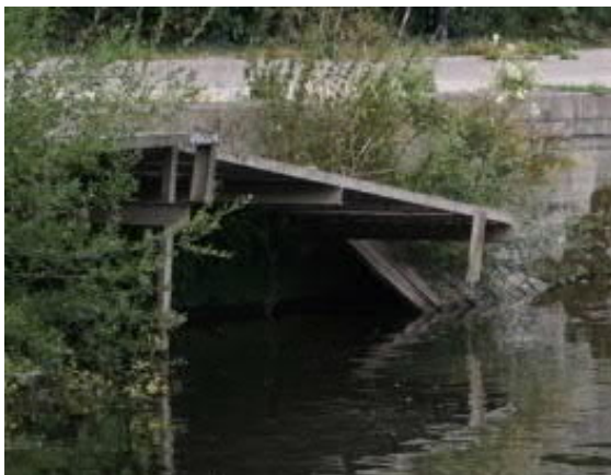
Figure 3-8 - Damaged Wooden Landing Stage Figure 3-9 - Concrete steps down to the river
