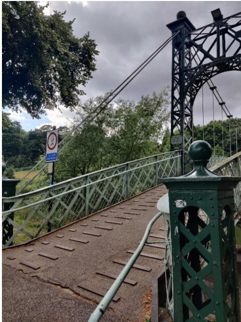
Figure 3-44 - The Quarry access to bridge
