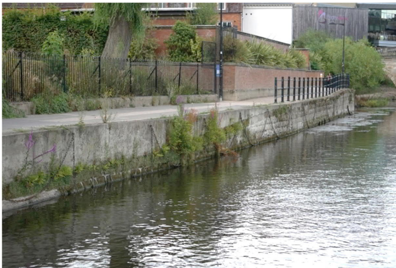
Figure 3-65 - Grab Chains along Water Lane
