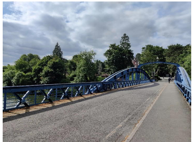
Figure 3-47 - Kingsland Bridge parapets
