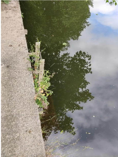
Figure 3-66 - Ladder at Mardol Quay
