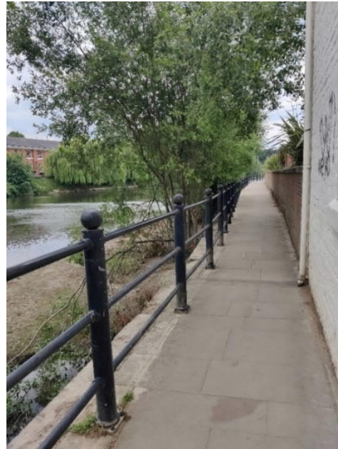
Figure 3-11 - Low river level behind barrier
