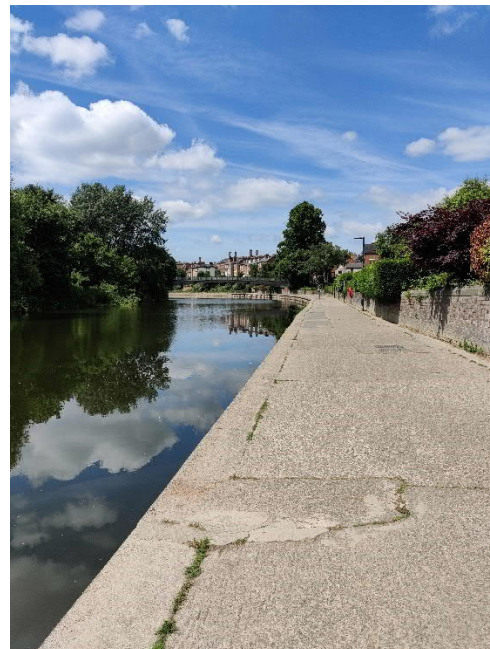
Figure 3-40 - Between Castle Walk footbridge and the weir
