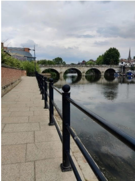
Figure 3-10 - Barriers near Welsh Bridge
